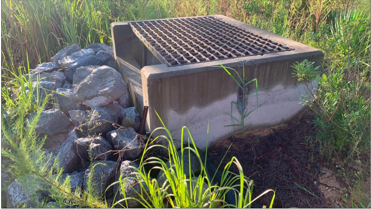
Figure 2.6.2 - Outlet Control Structure (2)
