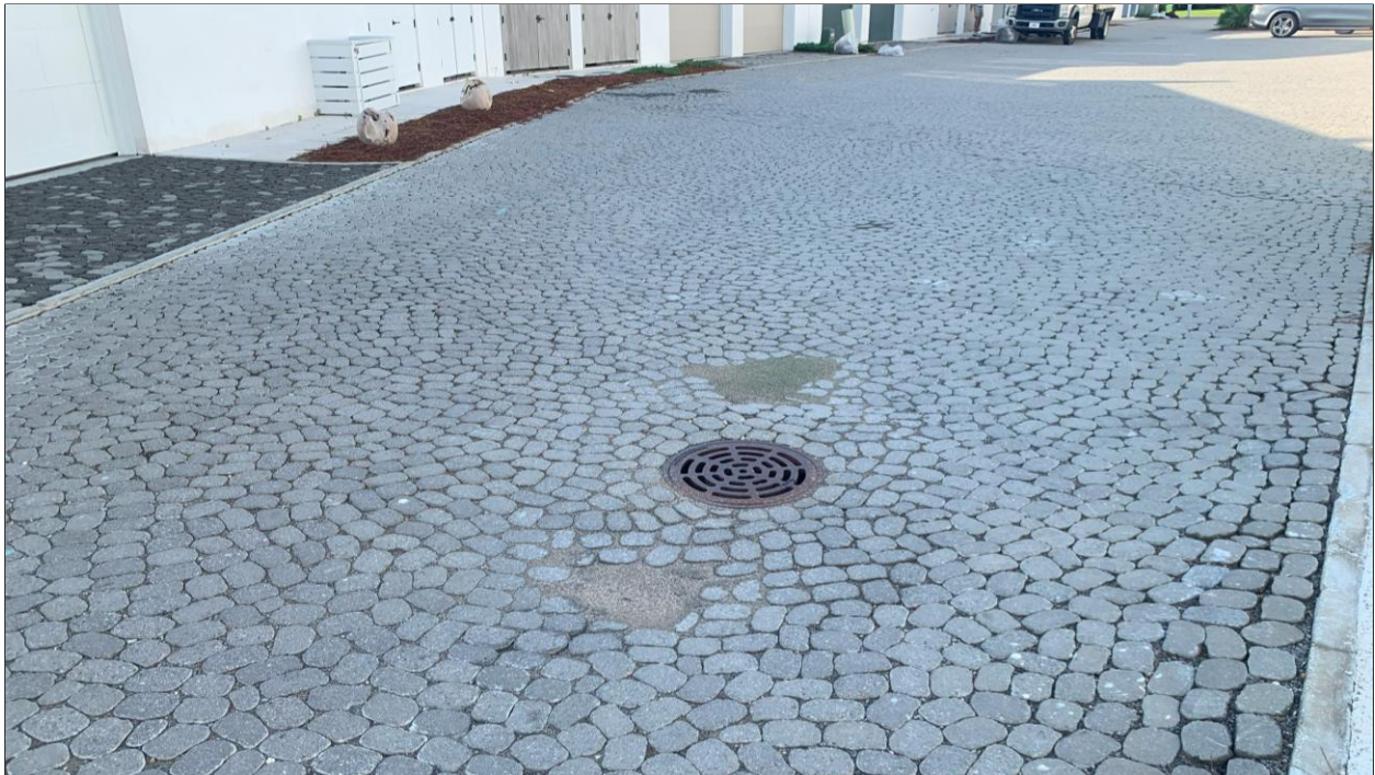
Figure 2.7.3 - Inlet to Exfiltration (2)
