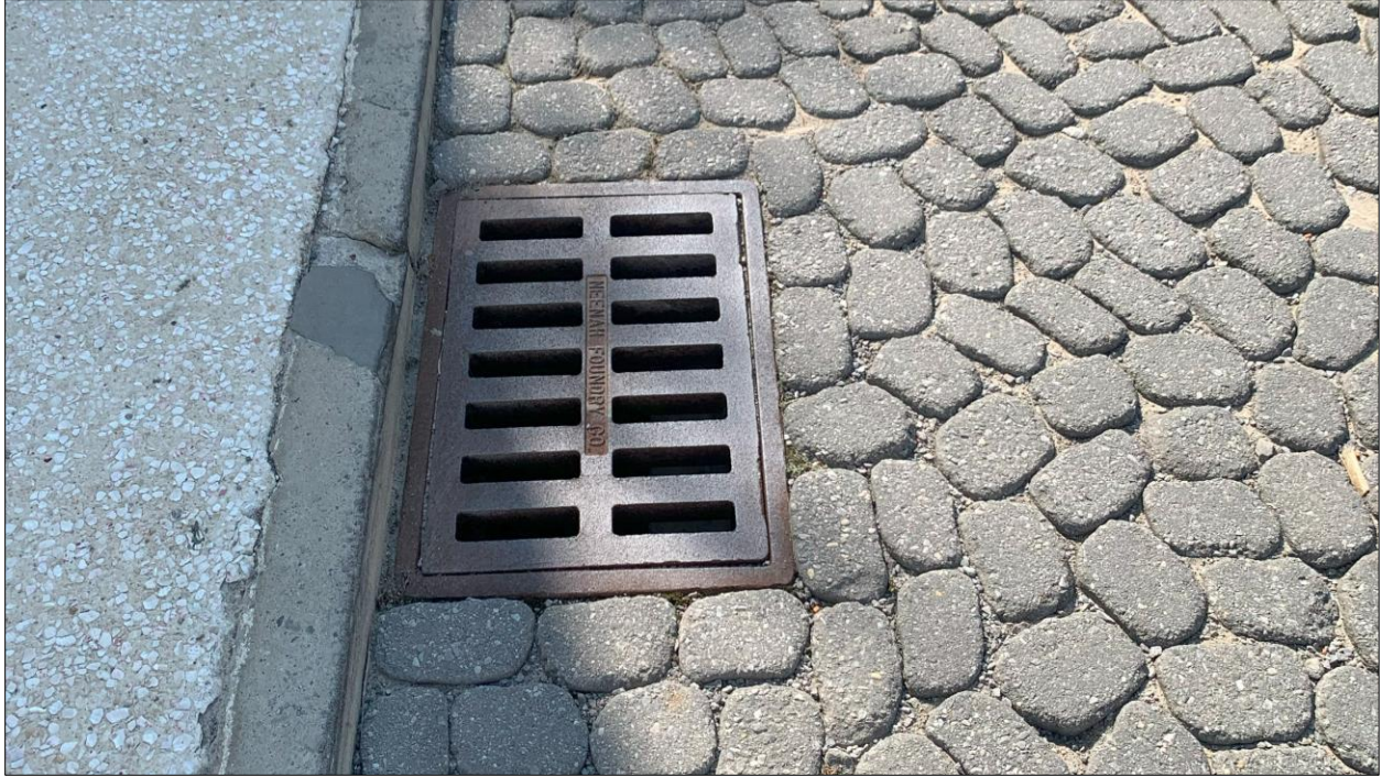
Figure 2.5.2 - Inlet to Exfiltration/Contech System (2)
