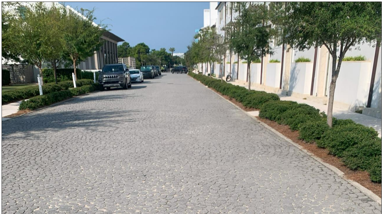
Figure 2.3.1 - Pervious Paver Roadway
