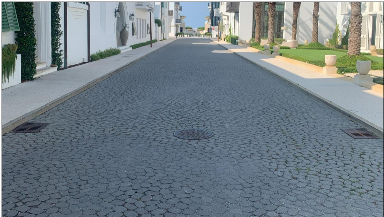
Figure 2.4.1 - Inlet to Exfiltration System (1)
