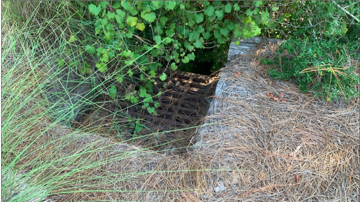
Figure 2.2.3 - Outlet Control Structure (2)
