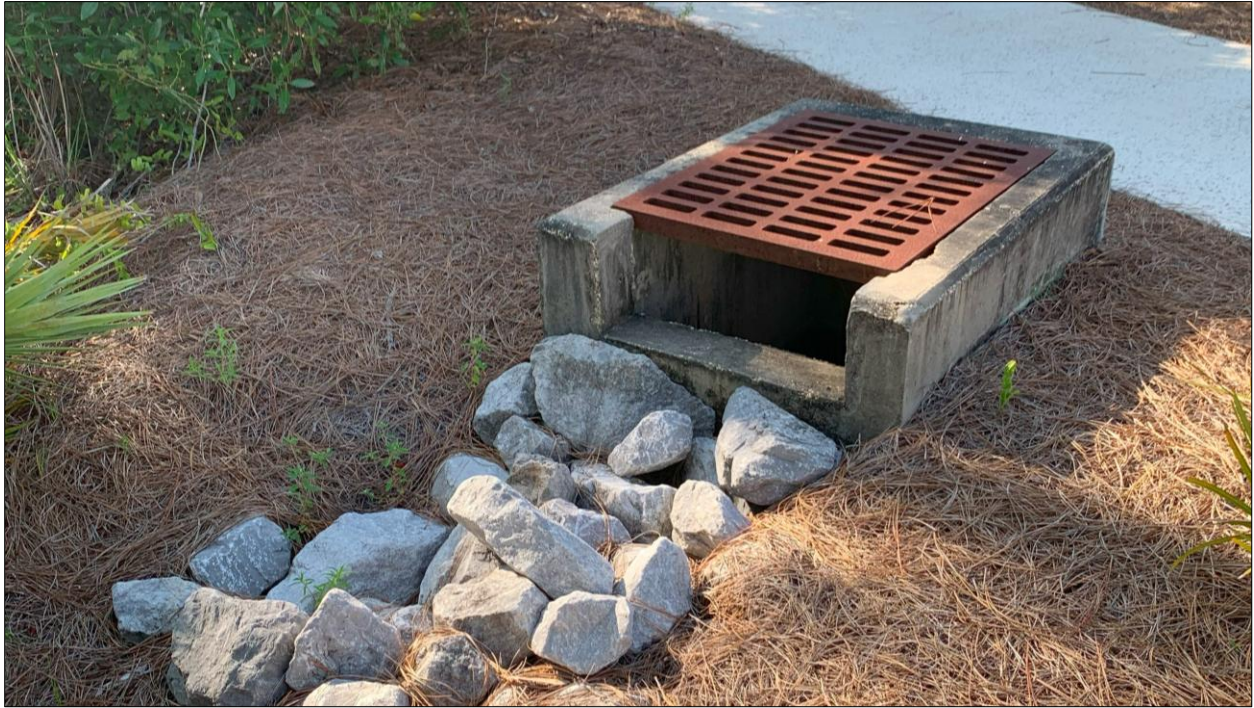
Figure 2.2.2 - Outlet Control Structure (1)
