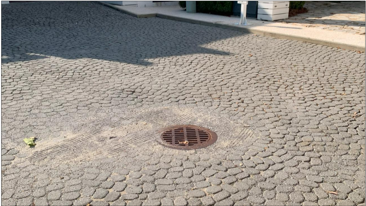
Figure 2.2.1 - Inlet to Exfiltration System
