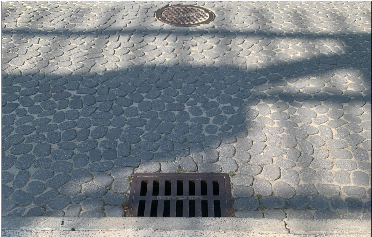
Figure 2.5.1 - Inlet to Exfiltration/Contech System (1)
