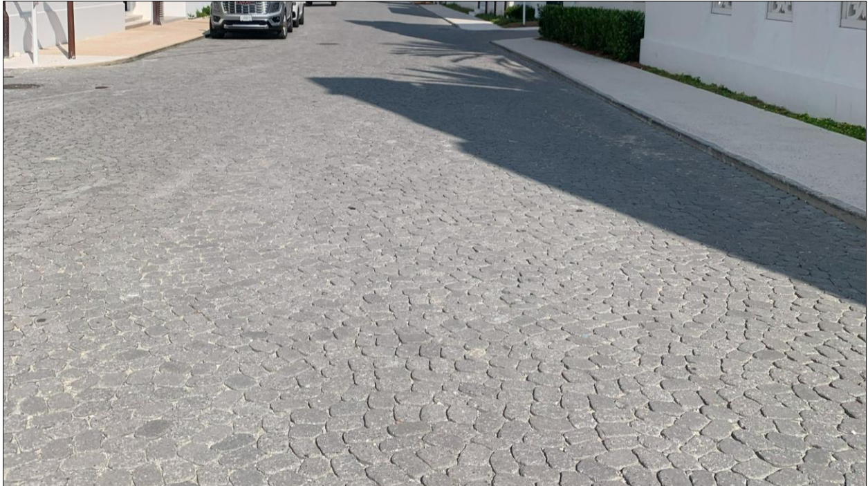
Figure 2.5.3 - Pervious Paver Roadway
