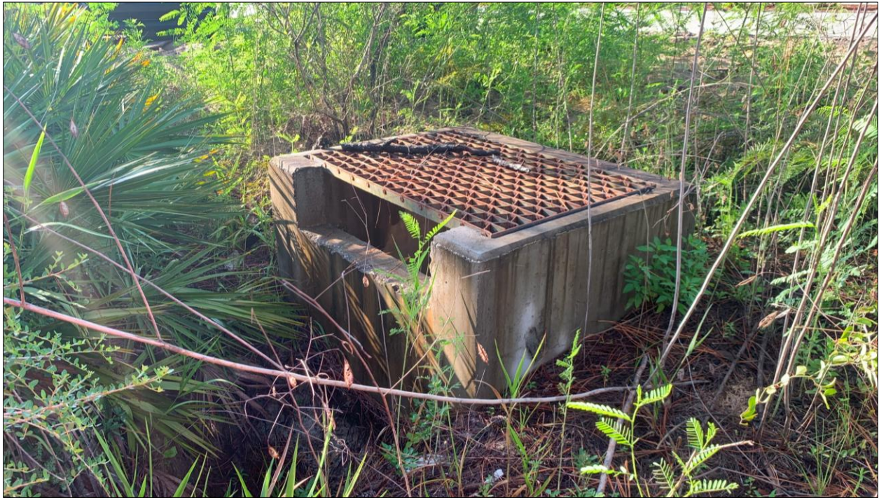
Figure 2.7.1 - Outlet Control Structure
