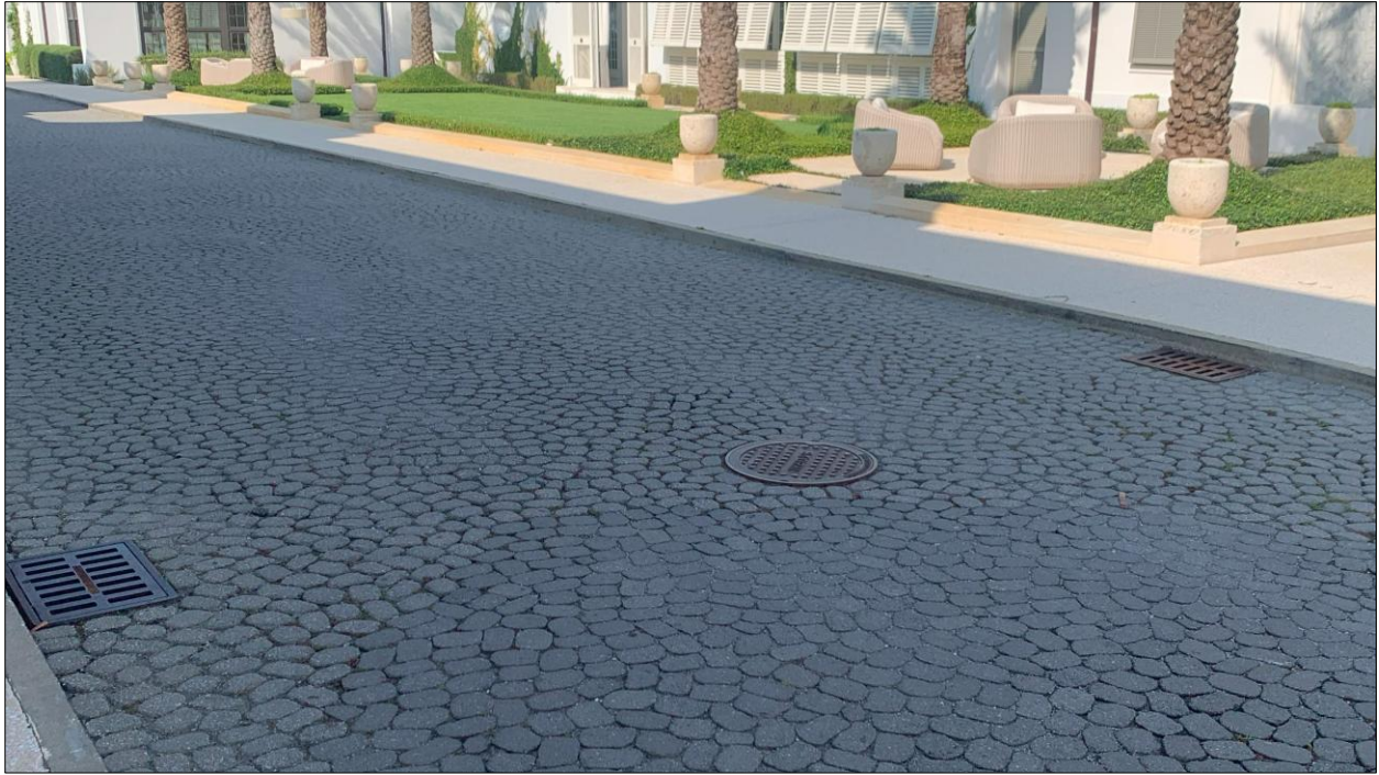
Figure 2.4.2 - Inlet to Exfiltration System (2)
