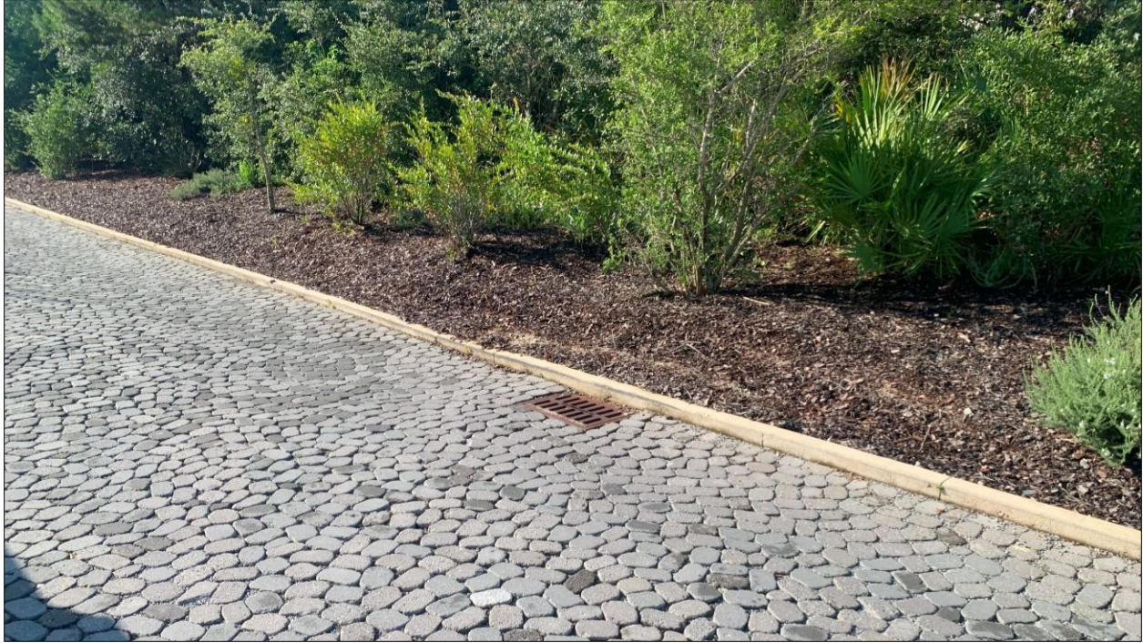
Figure 2.7.2 - Inlet to Exfiltration (1)
