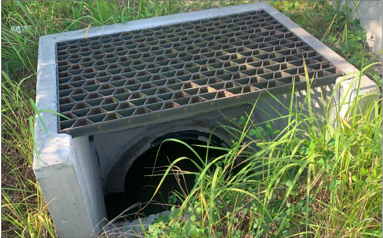
Figure 2.3.3 - Outlet Control Structure (2)
