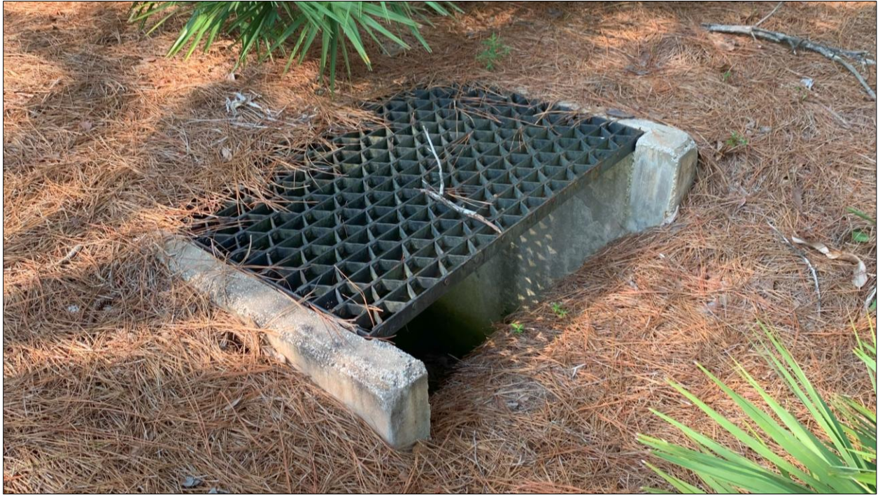
Figure 2.3.2 - Outlet Control Structure (1)
