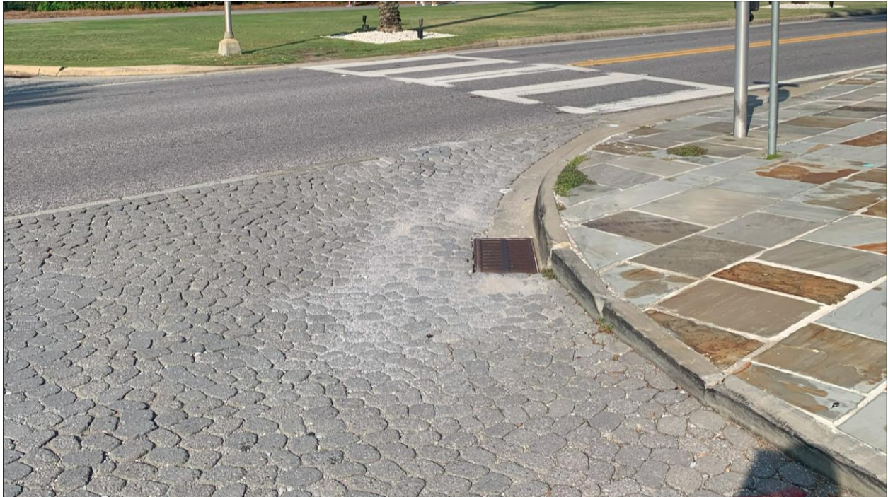
Figure 2.1.3 - Inlet to Exfiltration System
