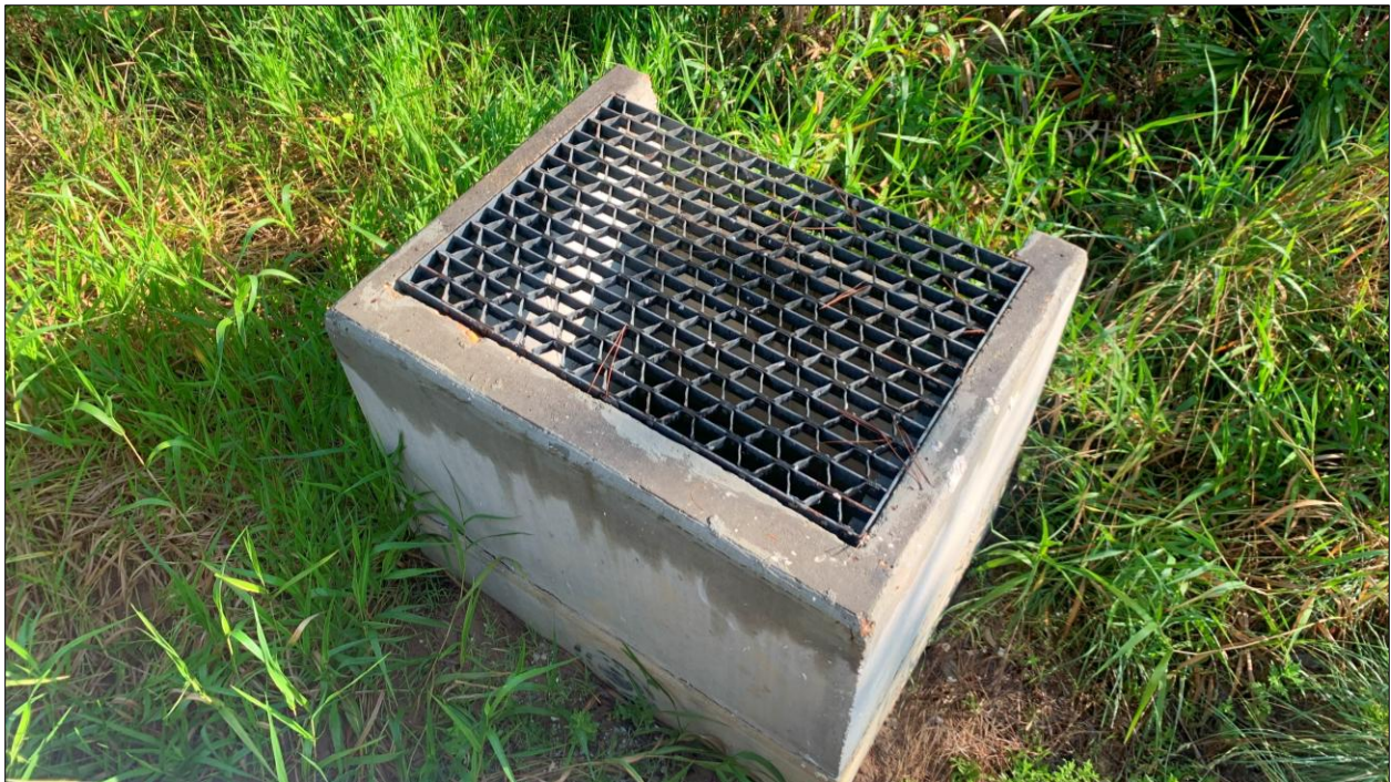
Figure 2.6.1 - Outlet Control Structure (1)
